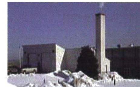
Darby public school biomass heating plant.
